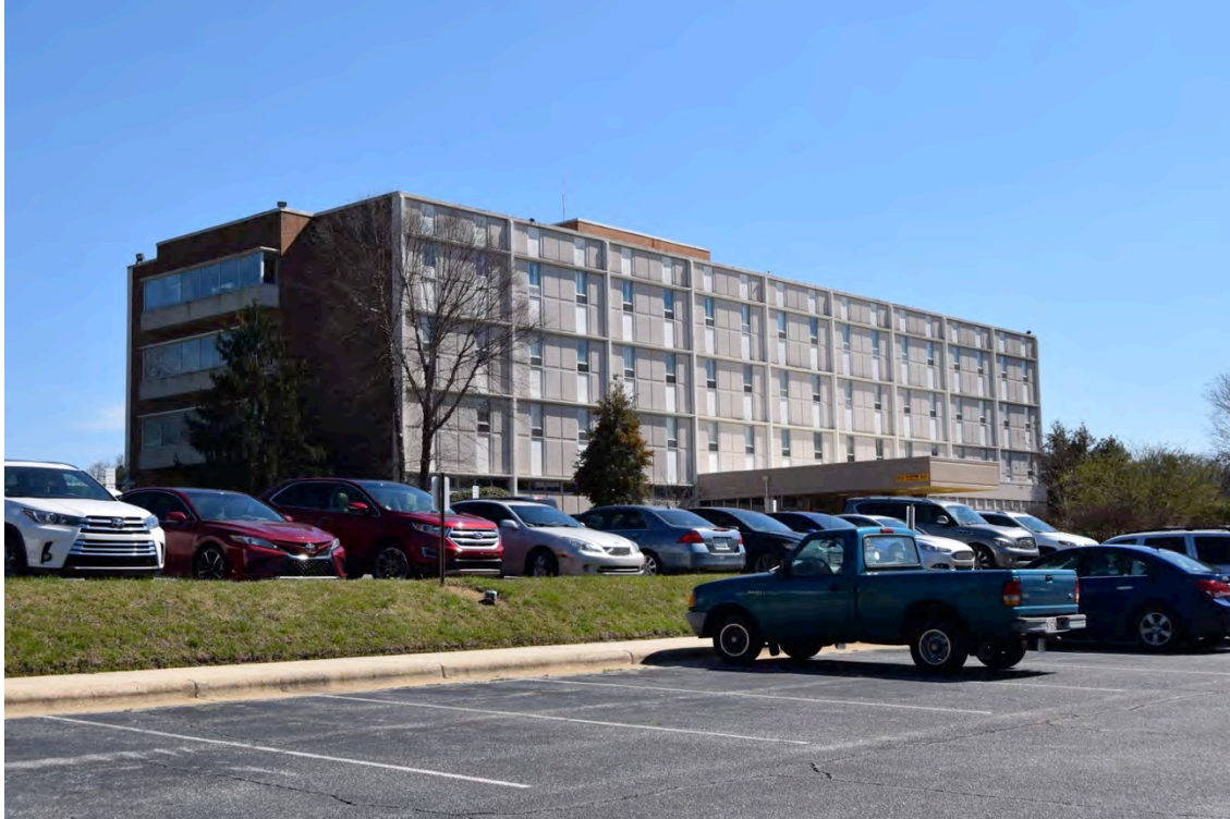
West elevation and façade, L. Richardson Memorial Hospital II (GF6065), view E
