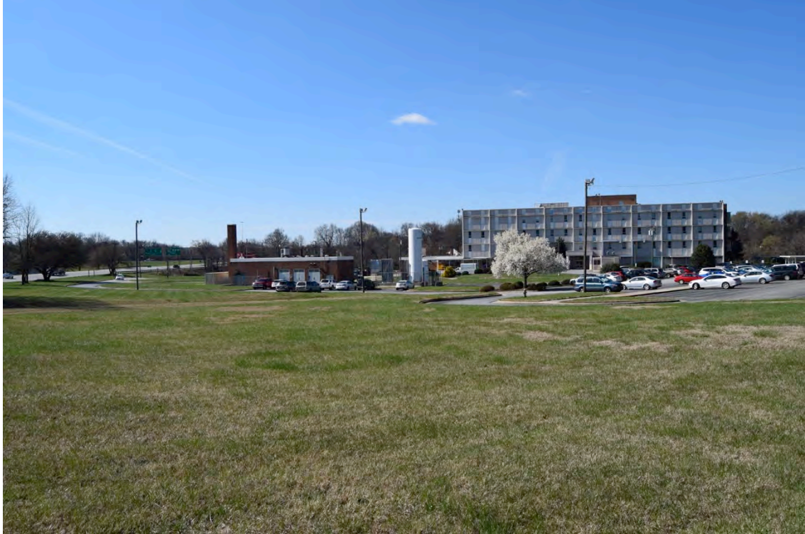
Rear view, L. Richardson Memorial Hospital II (GF6065) from parcel edge near roadway. View W.
