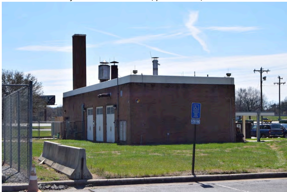
Rear and west elevation, power house, view SE
