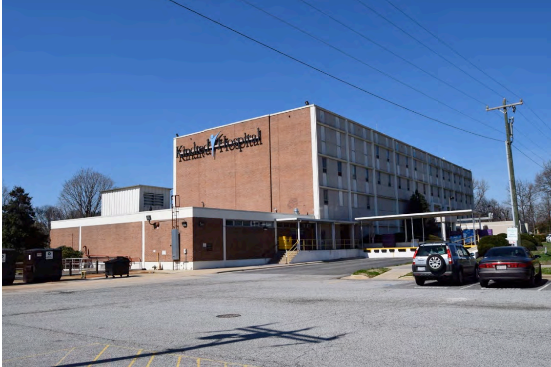
East and rear elevations of L. Richardson Memorial Hospital II (GF6065), view NW
