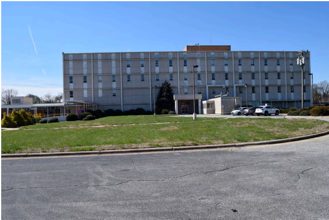
Rear elevation L. Richardson Memorial Hospital II (GF6065), view SW
