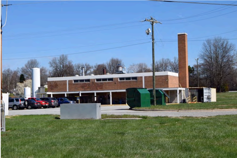
Façade and east elevation, power house, view N
