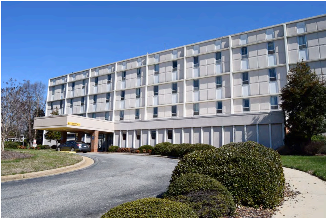
Façade view showing front entrance and façade wing, view NE.
